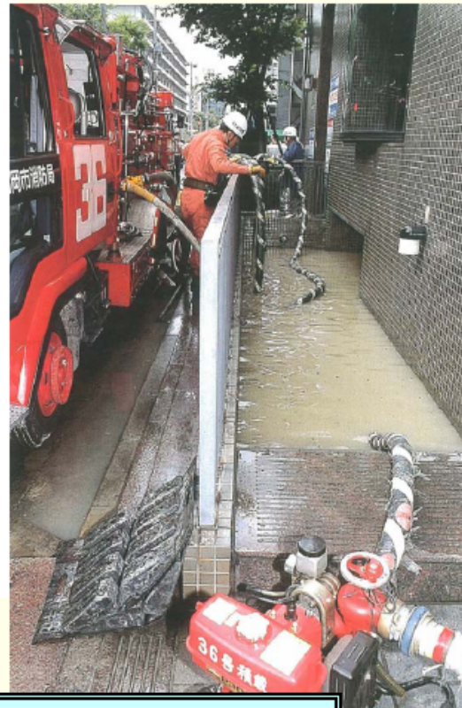
Inundation of basement during Fukuoka Flood of June 1999
