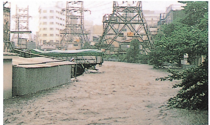
Kanda River in flood during Typhoon No. 11 in 1993
