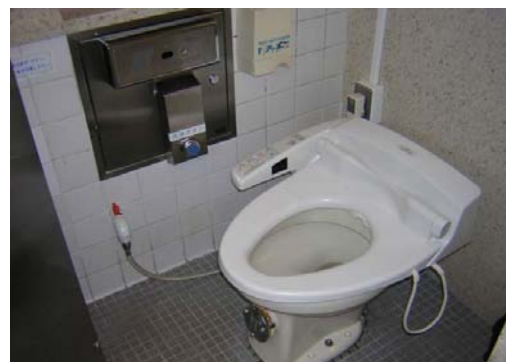
Figure 6. Existed Toilet in Moriya service area.
