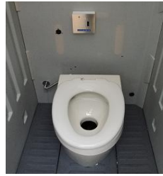
Fig. 2: Water recycling urine-diverting toilet
