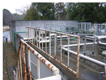
Fig. 8: Domestic wastewater treatment facility in Minori service area
