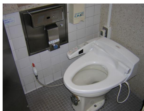
Figure 6. Existed Toilet in Moriya service area.
