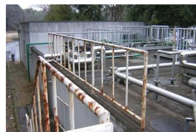
Figure 6. Domestic wastewater treatment facility in Minori Service Area
