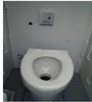
Figure 2. Water recycling urine-diverting toilet (Reinforce,2010)
