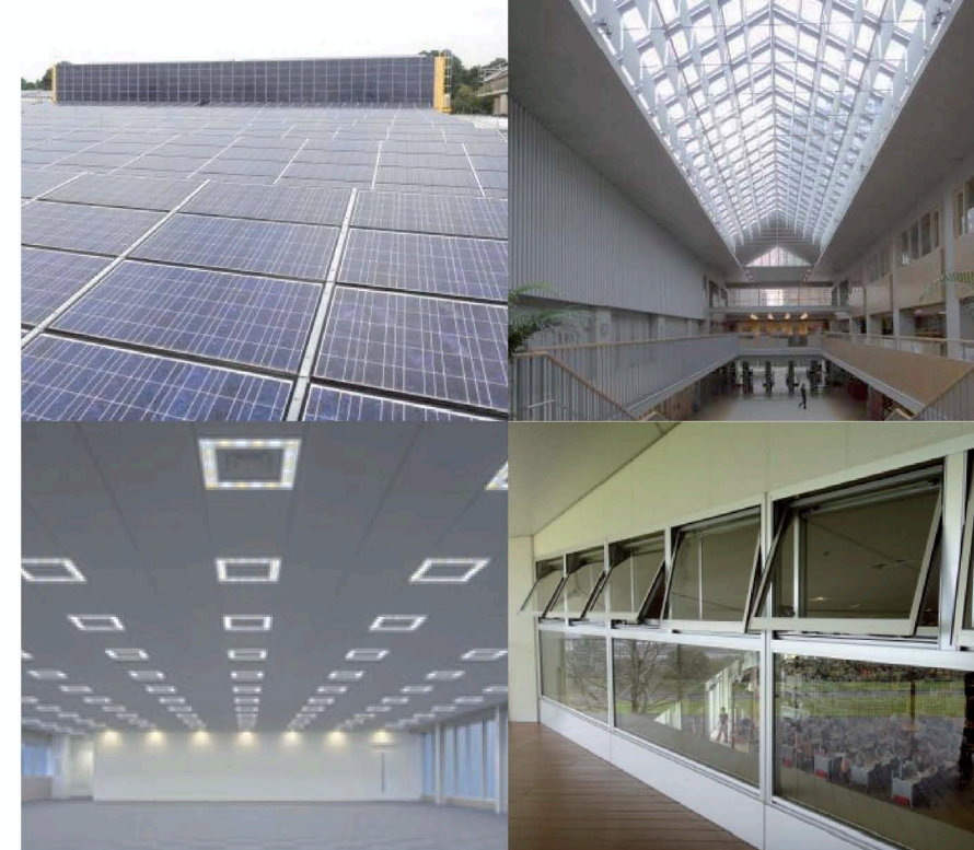
省エネ、再エネの最新技術 | (左上より右回りに) 太陽光パネル発電、自然採光利用、自然換気システム、LED照明 State-of-the-art energy-saving and energy-recycling technologies | Clockwise from top left, Power generation by solar panels, Natural lighting use, Natural ventilation system, LED lighting
