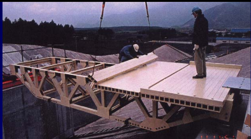
床版铺装 Floor Slab Construction
