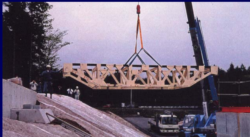
Block Erection using 12ton Crane
