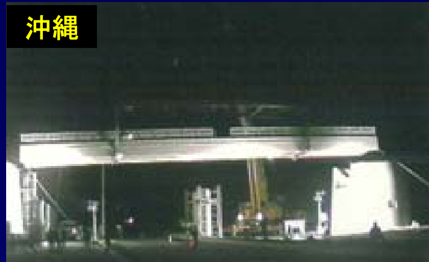
Large Block Erection at Site
