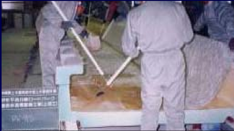
Hand Lay-up of Main Girder
