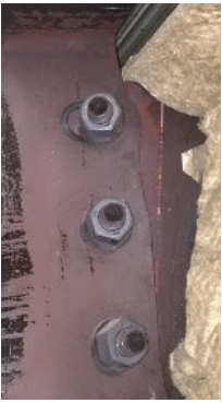
Photo 5 Bearing Photo 6 Bearing deformation of lower flange in contact with gusset plate
