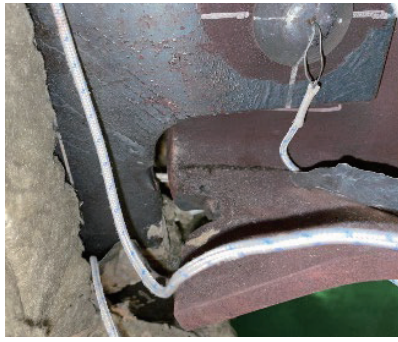
Photo 5 Bearing Photo 6 Bearing deformation of lower flange in contact with gusset plate
