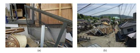
Fig. 9. Wooden houses in the Kumamoto earthquake in 2016. (a) Connection failure; (b) collapsed houses.
