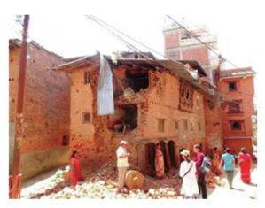
Fig. 1. Unreinforced masonry building damaged in the Gorkha earthquake in 2015 [3].
