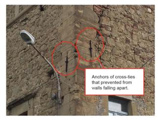
Fig. 4. Surviving masonry building with cross-tie reinforcement in the Amatrice earthquake.
