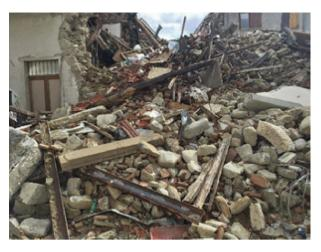
Fig. 3. Collapsed masonry buildings in the Amatrice earthquake in 2016.
