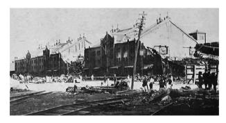
Fig. 5. Masonry buildings damaged in the Great Kanto Earthquake in 1923 [5].
