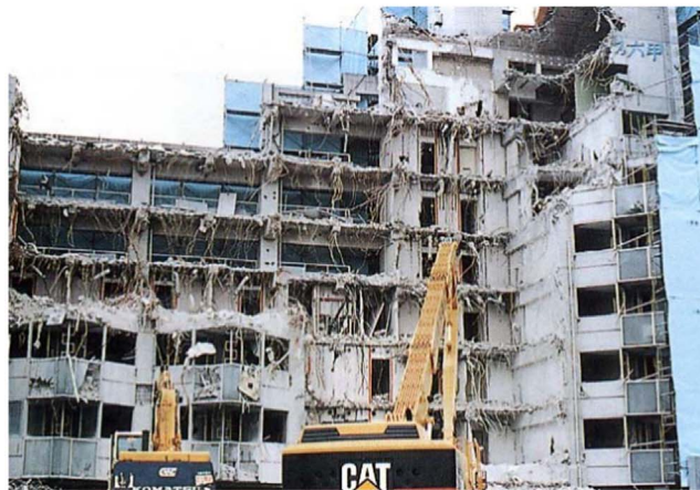
(b) Demolished building
